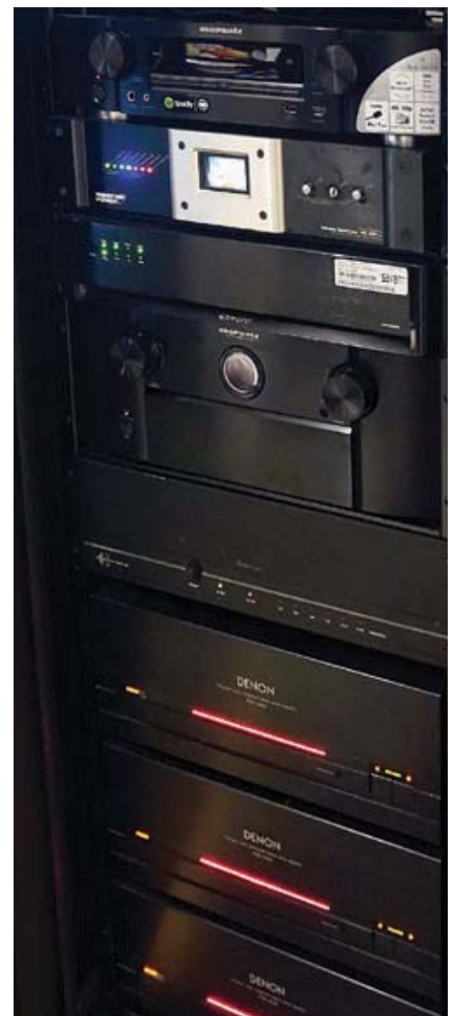
Neatly powering the home automation system is a selection of gear housed in a Middle Atlantic AV rack in the basement, including everything from Bell Fibe PVRs, to a pre-amp, AV receiver, amplifiers, Savant control system with pro host, WirePath DVR, and other connected devices.
